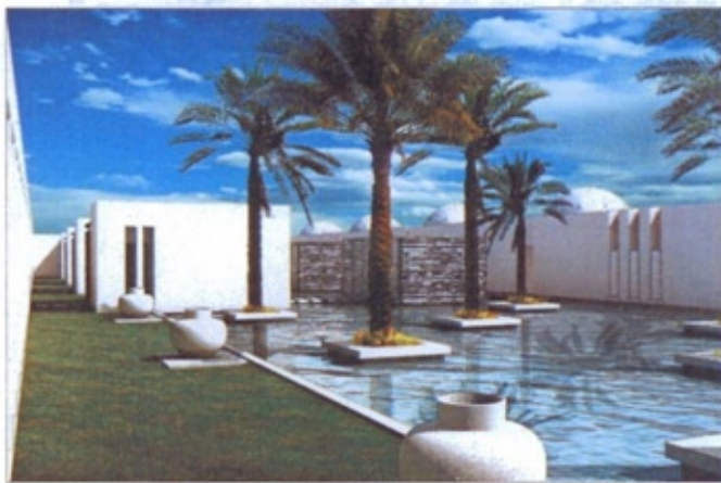
Set for completion by the end of 2010, The Malkai is located about 50 kilometres from Muscat in the Al Batinah region
